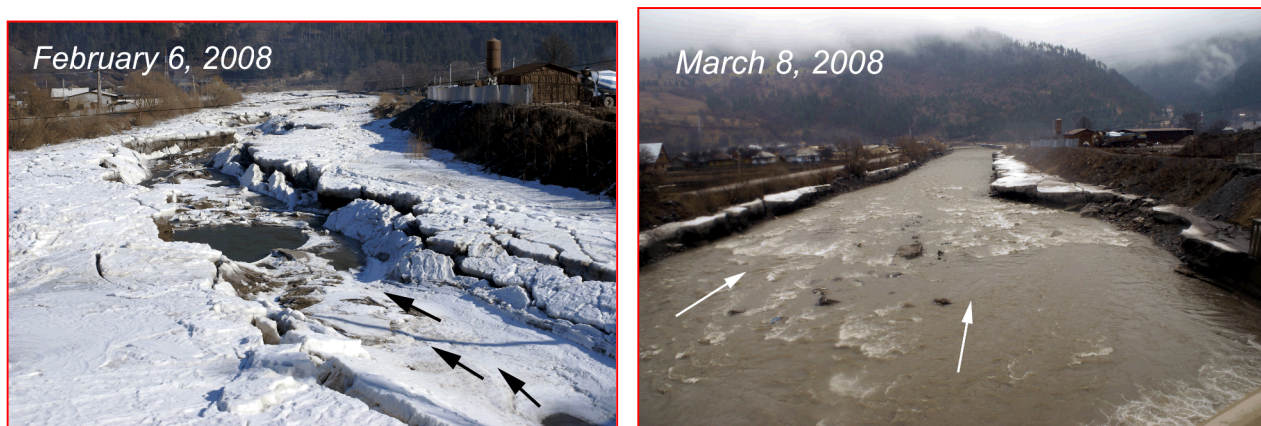
Fig. 4. Bistrita river channel downstream Topolicești bridge filled by freezep jam (February 6, 2008) and almost open (March 8, 2008).
